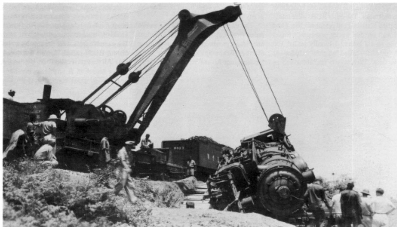
Basye's sabotaged-caused train wreck - Courtesy of John Daoutis
